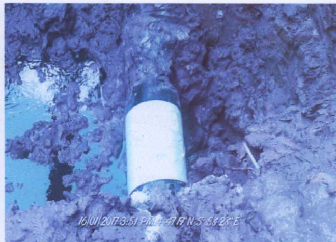
Figure 2: Coned after repair on the Pipeline .
